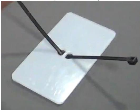
3. Locate the Under Tile Plates between the breaks in the tile with the ends of the cable tie sticking up through the tile. Slide each plate under the tile in the locations as shown.
